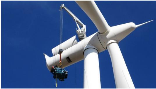
Figure 3.13: Liftra self-hoisting crane
