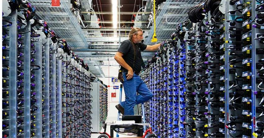
Figure 3.2: Exchange of a server
