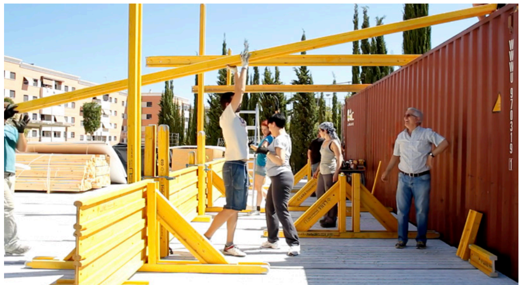
Construction of the dining room, photograph, 2017.
