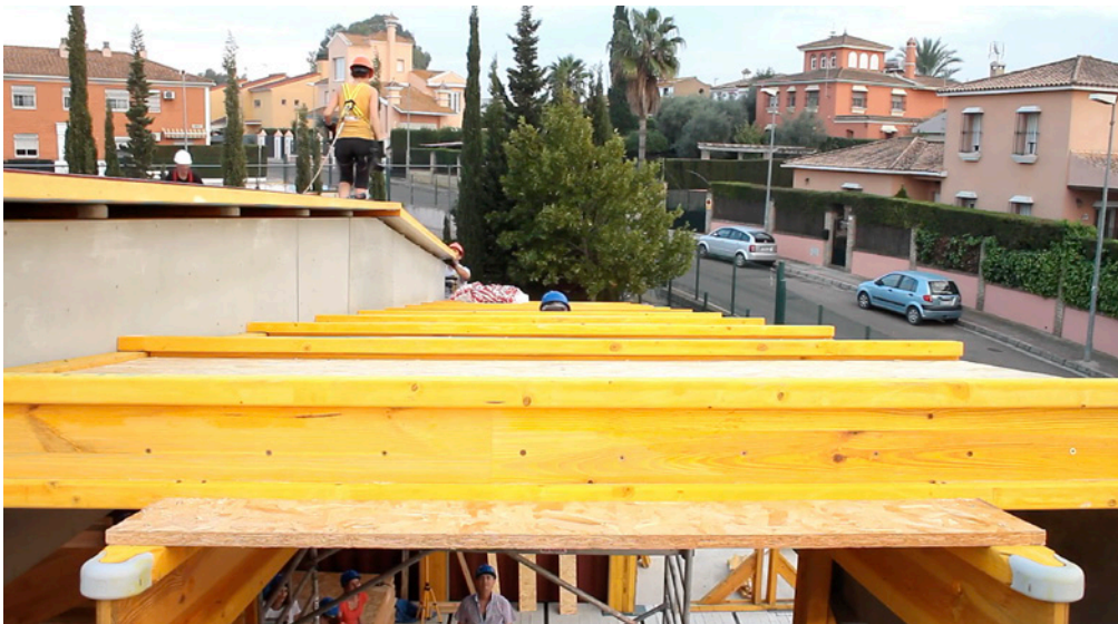
The construction of the roof of the dining room
