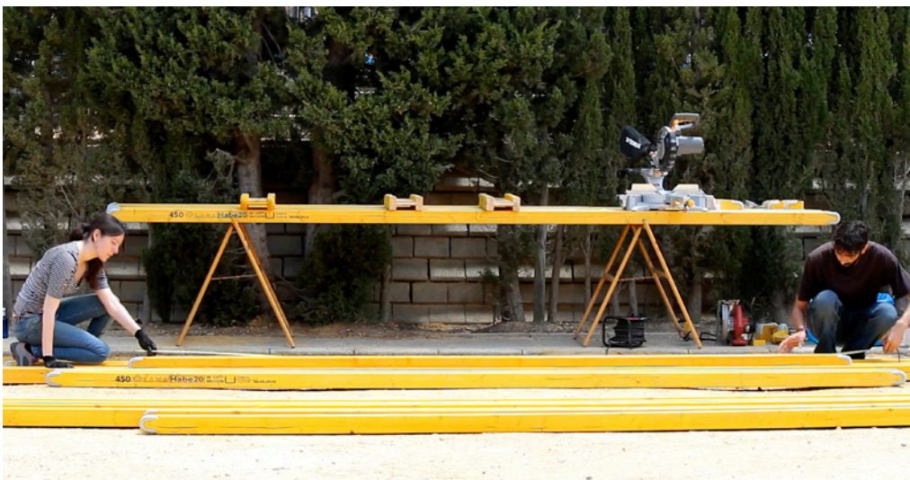
Construction of the dining room, photograph, 2017.
