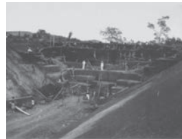
The making of railroad tracks around Purwakarta.
