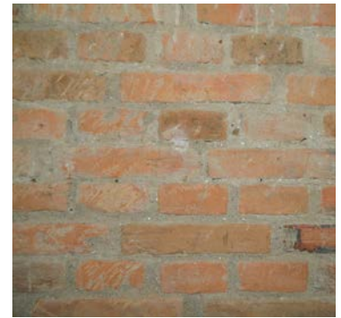
3. Part of the brick masonry wall of the building
