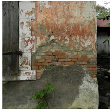
2. Arrangement of bricks in the corner
