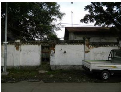
1. Front Wall, South Elevation.
