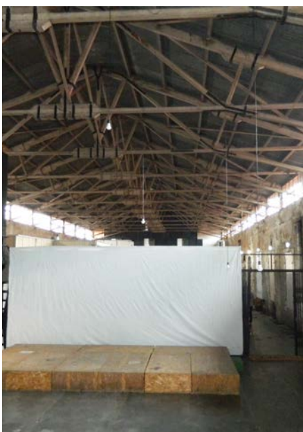
example of a building with visible roof structure and an open plan
