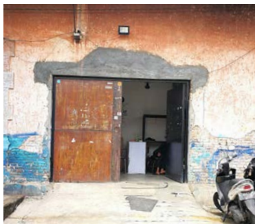
4. Some warehouses have areas cut out for this new bigger door type.
