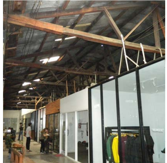
Existing roof structure with additional steel elements
