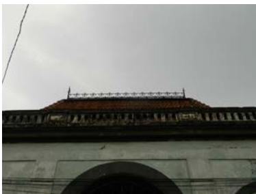
Classical architectural details: balustrades, pilasters & acroteria, with a prominent display of richly detailed clasps, brackets and supporting consoles
