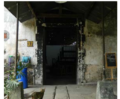
3. Door type used for Spatial. Ventilation space on top of the door.
