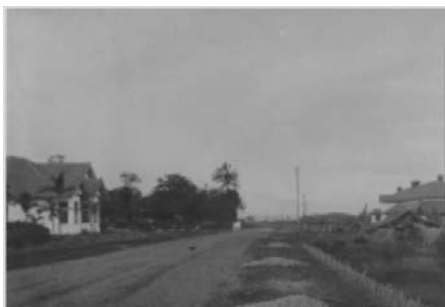
Housing construction on Jalan Riau which is still quiet.
