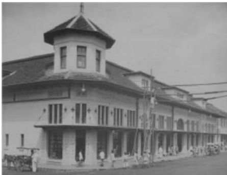
Busy people were installing street lighting in front of the new De Vries Shop.
