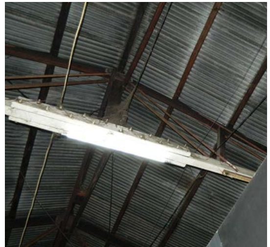
Existing roof structure with additional steel elements
