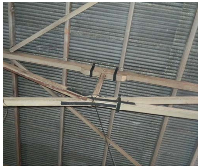
The different timber elements are connected with cast iron joints.
