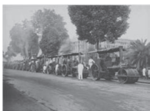
The “Stoomwals machine” is used to pave the streets of “Gemeente Bandung”.
