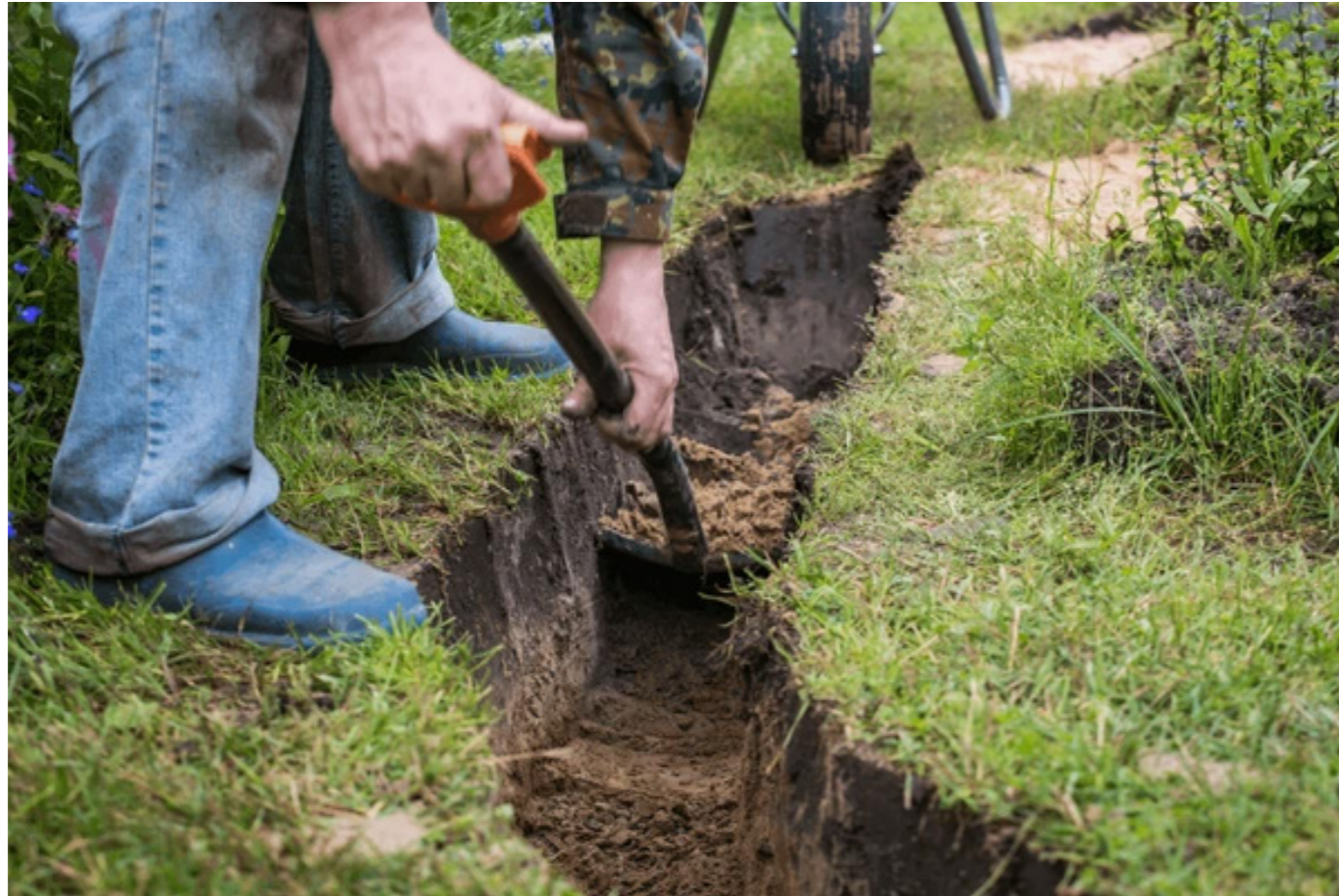
Source: Digging Trench, shutterstock, Ilia Baksheev
