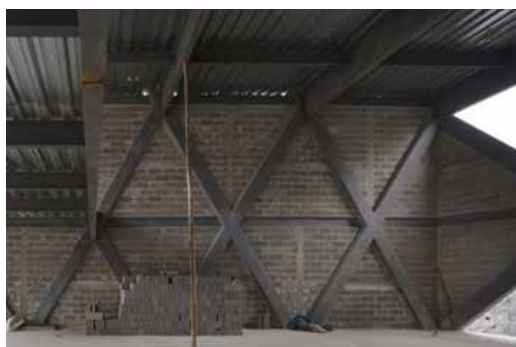
Figure 40: Local private and social buildings with concrete blocks. Source, Cabezas, 2018
