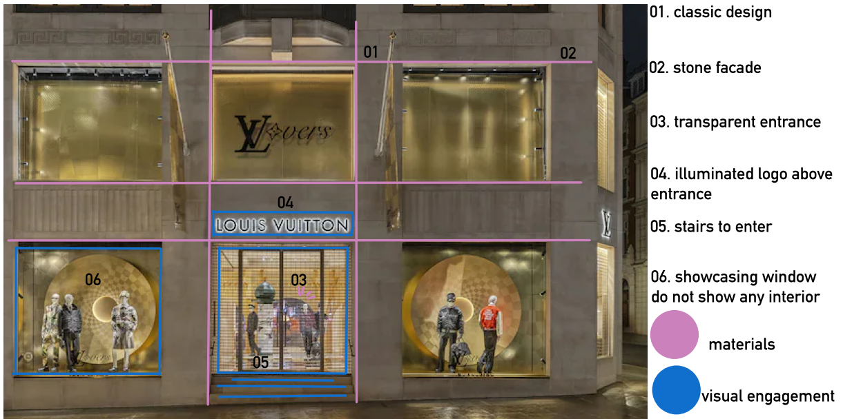
Figure 33. Louis Vuitton New Bond Street exterior at night. [façade analysis]
