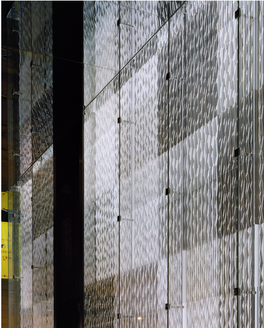
Figure 17. Louis Vuitton facades metal envelope. [stainless steel zigzag blades]
