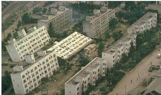
Figure A.20: Rigid body rotation of several residential buildings as a result of liquefaction due the 1964 Niigata Earthquake.
