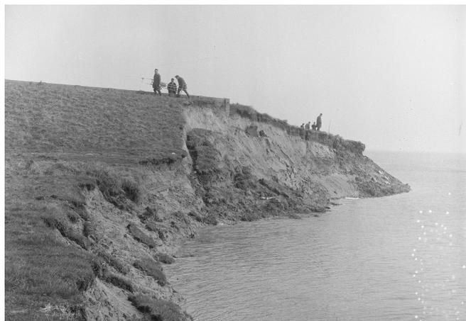
Figure A.16: Flow failure near Kats in Zeeland, the Netherlands in 1966. From <https://www.nationaalarchief.nl/>
