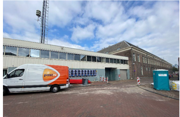
Old and new volume south facade (own image).
