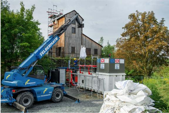
**Figure 3-3:** Separation and injection container, and entrance to mineshaft
