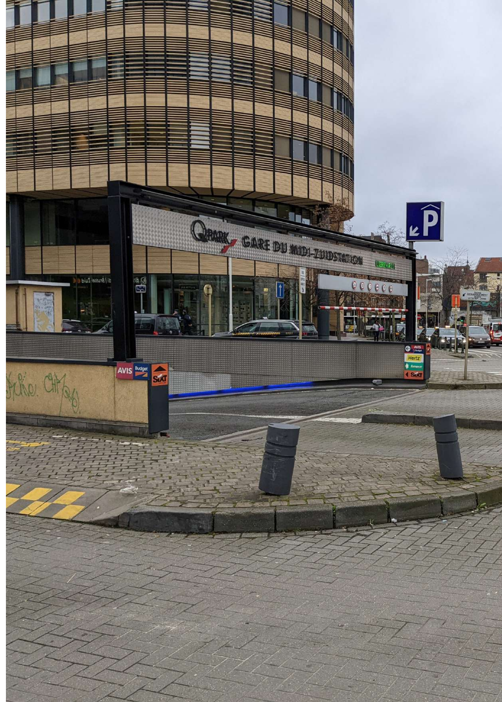
Figure 3.5 (Right): The Parking garage of Brussels-South
