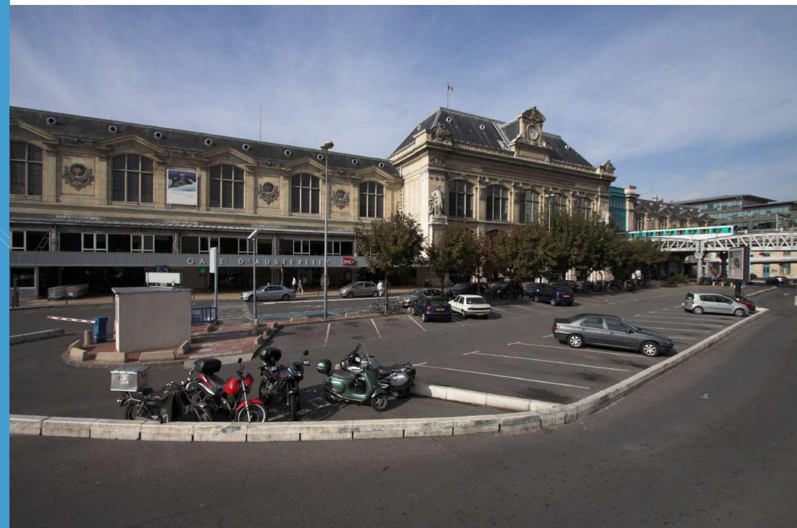
Figure 8.1: The main entrance of Paris Austerlitz. Source: Wikimedia commons
