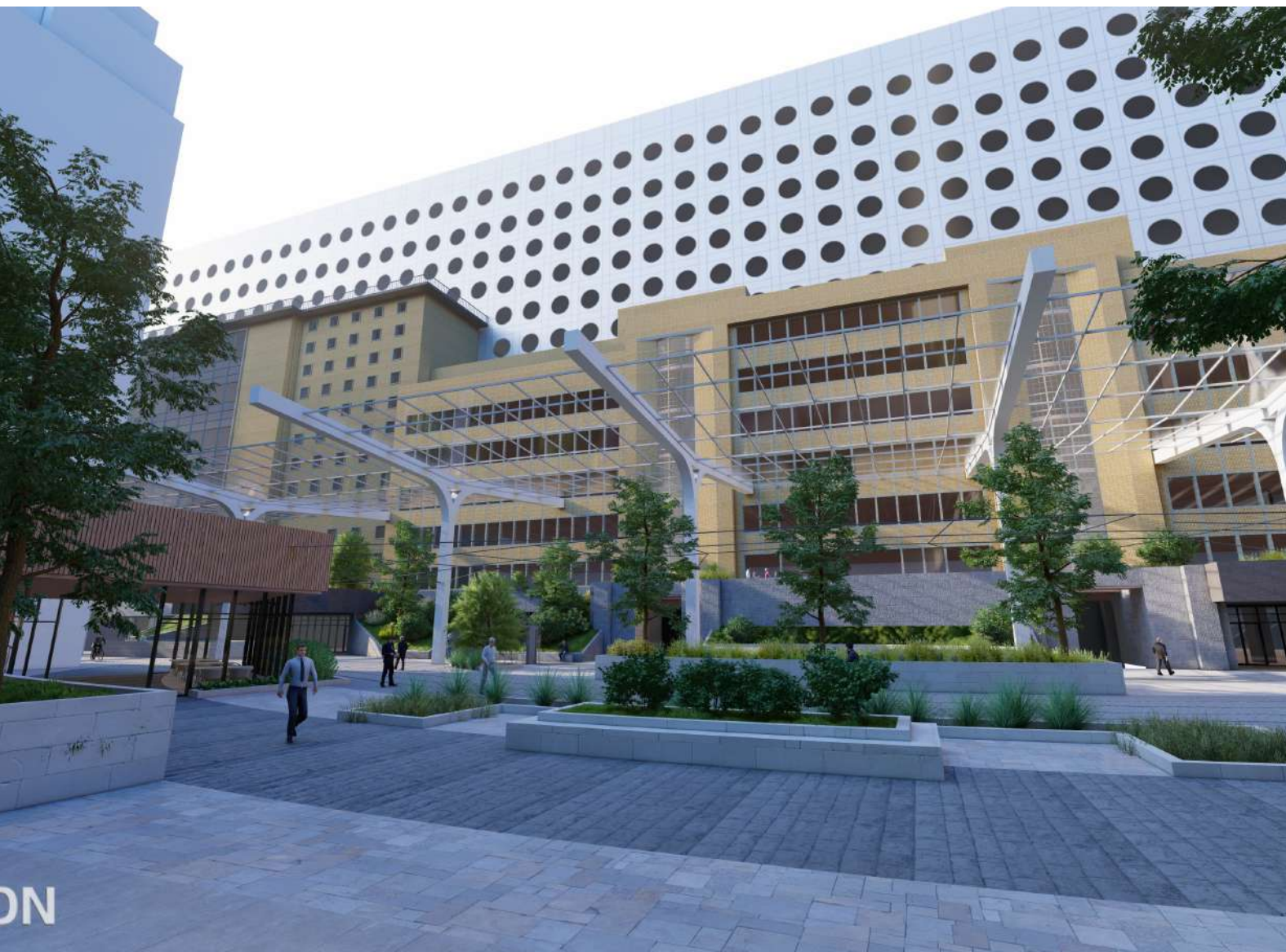
Figure 16.8: The roof above Avenue Fonsny
