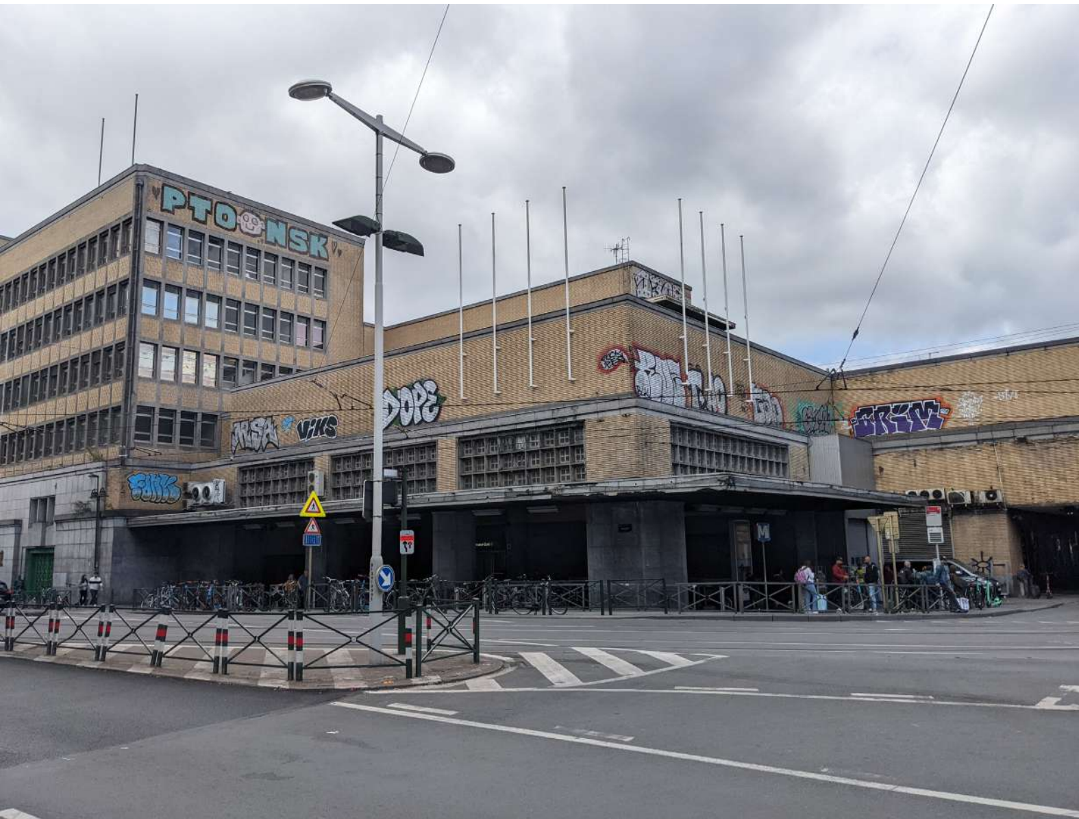
Figure 11.6: Avenue Fonsny Covered Street Entrance
