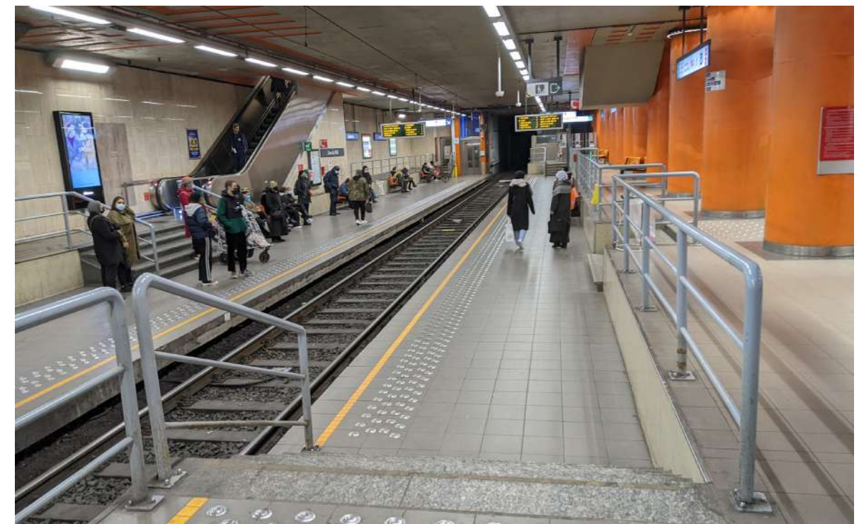
Figure 9.4: The current pre-metro platform underground.
