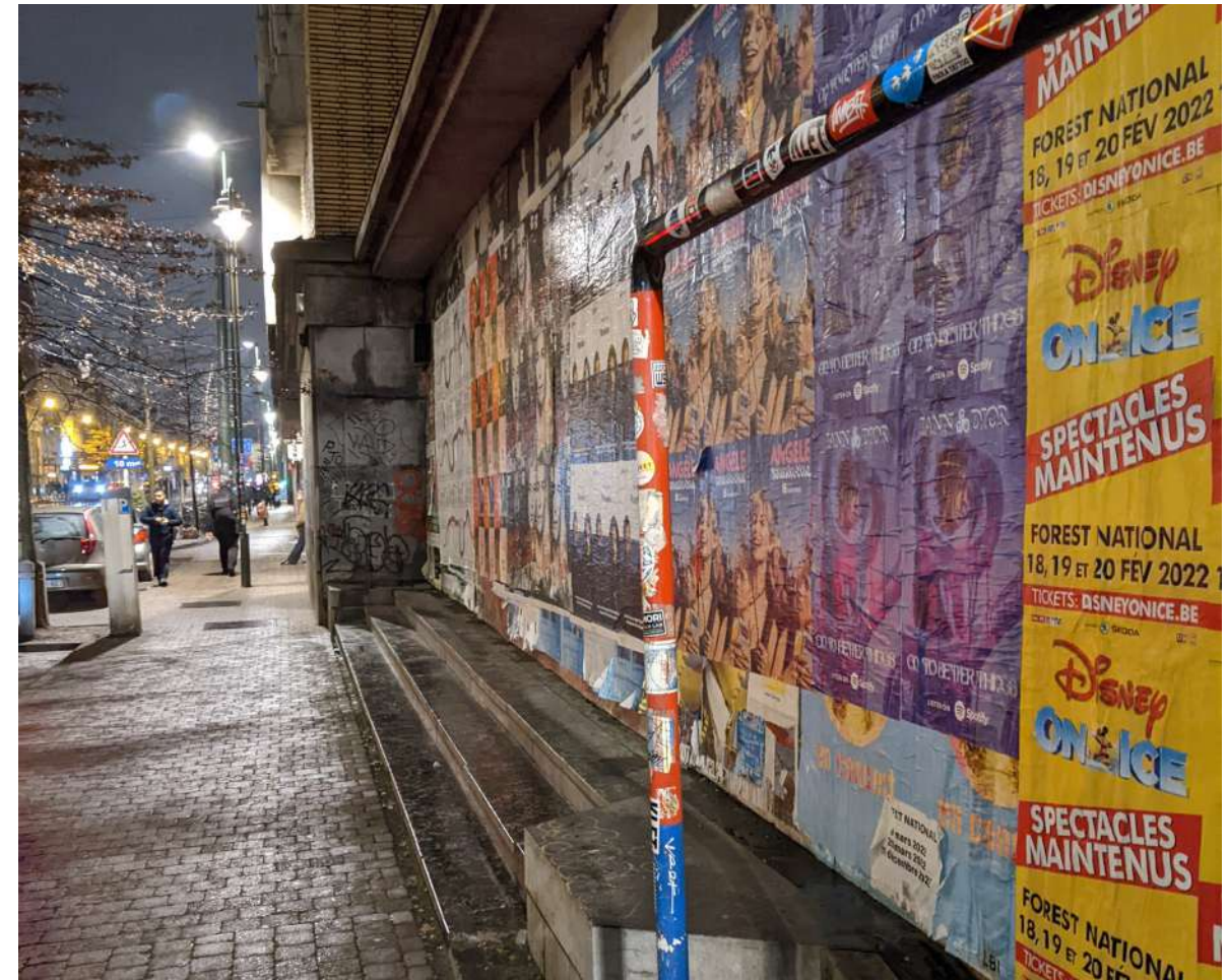
Figure 4.3: The closed entrance at Brussels-South, blocked off with wooden panels
