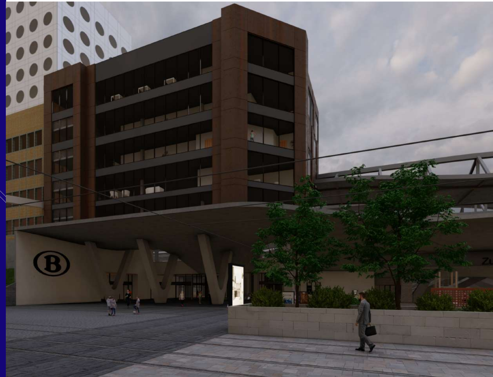
Figure 18.1: The Extension of the Post Office Building
