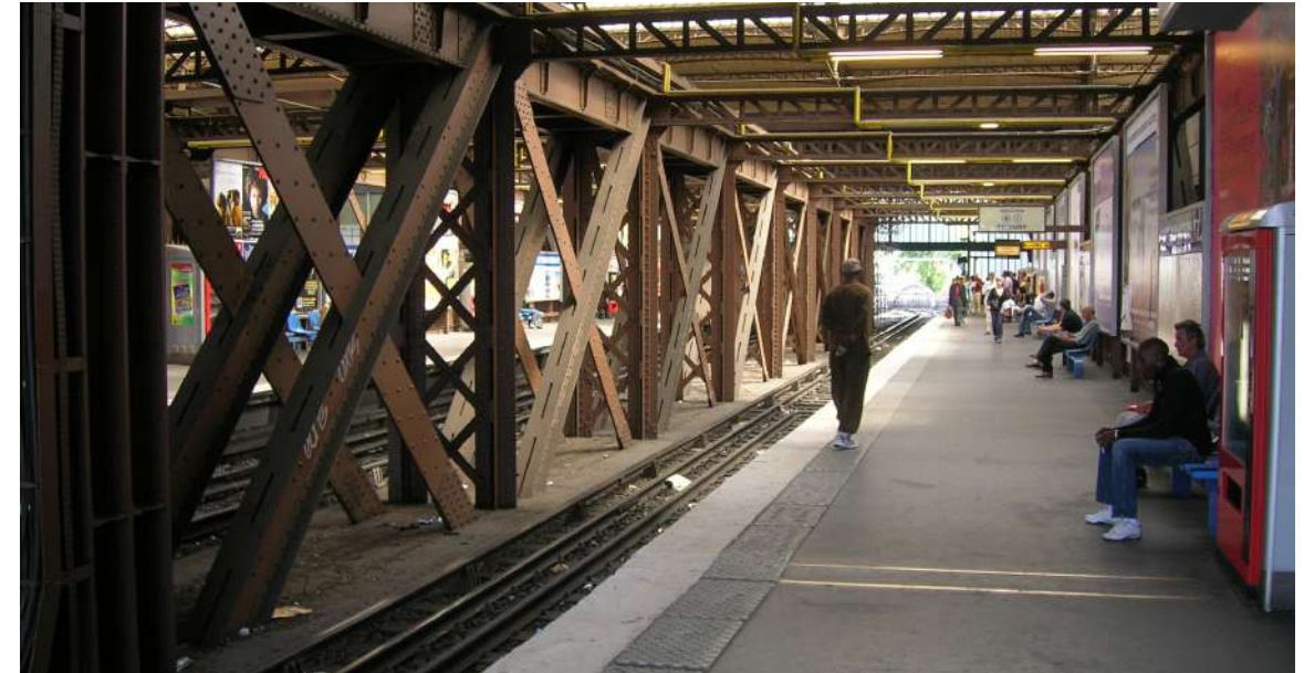
Figure 8.16: Upper Metro Station. Source: Wikimedia commons
