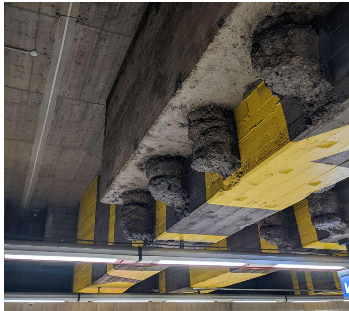
Figure 15.2: The Foundation pillar of the existing rail bridge.
