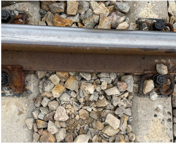
Figure 17. Ballast layer in the field at railway line section K17+700.
