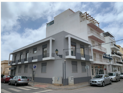
Figure R3. Picture of buildings on plots H and I
