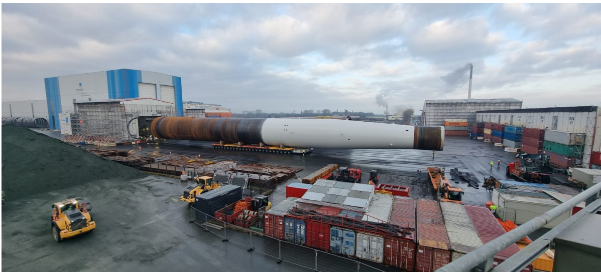
Figure 36: Site move at Steelwind
