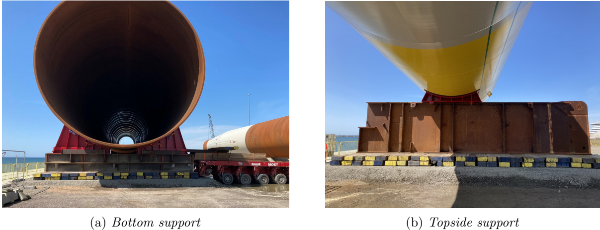
Figure 8: Temporary steel supports on quayside
