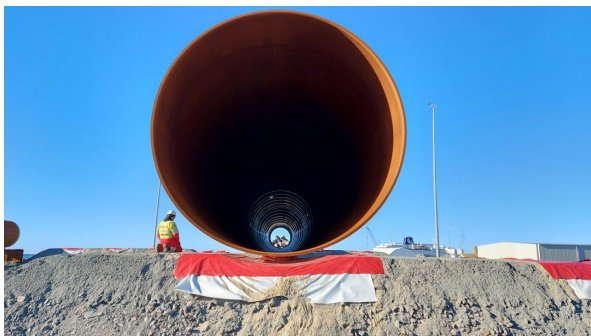
(a) Monopile laydown
