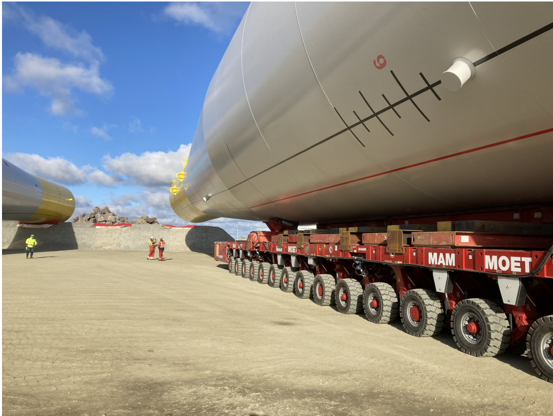
Figure 42: Monopile transport with SPMT
