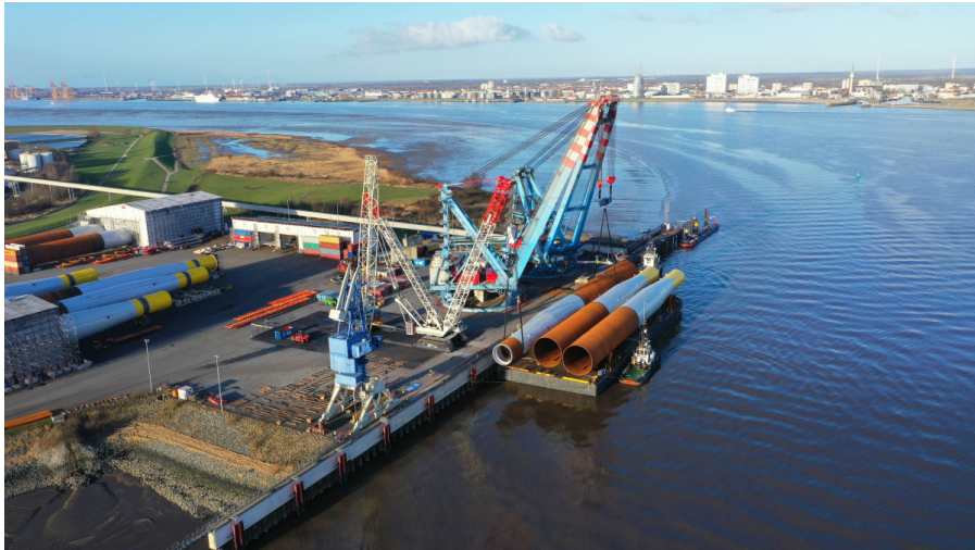
Figure 37: Load out at production facility (Dillinger, 2022)
