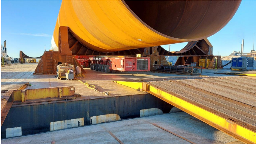
Figure 40: Seafastening grillage and RoRo ramps
