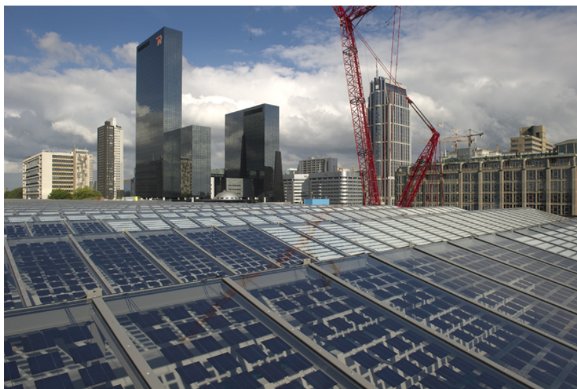
Figure 1.4: Building integrated solar panels in the glass roof of the Rotterdam Centraal station. Retrieved from [3].
