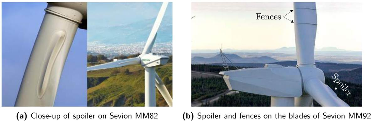
**Figure 2.3:** Spoilers installed on Sevion MM82 and MM92 wind turbine blades
