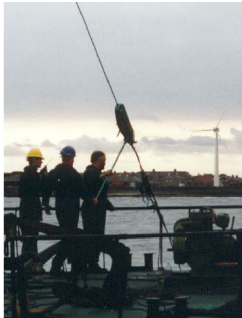
Figure 1.6: Strain gauge calibration by anchor, cable, winch and load cell, operated from a barge next to the wind turbine [14].
