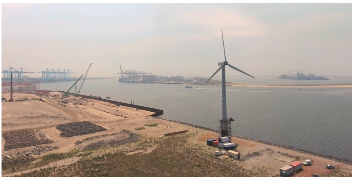
Figure 2-1: Aerial view of the DOT500 on the Maasvlakte II, The Netherlands. The DOT500 proved the ability to control the rotor speed of the wind turbine through the line pressure [28].
