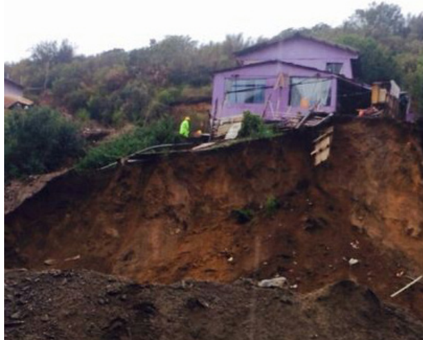
Landslide in Valparaíso (Caballero, 2014)
