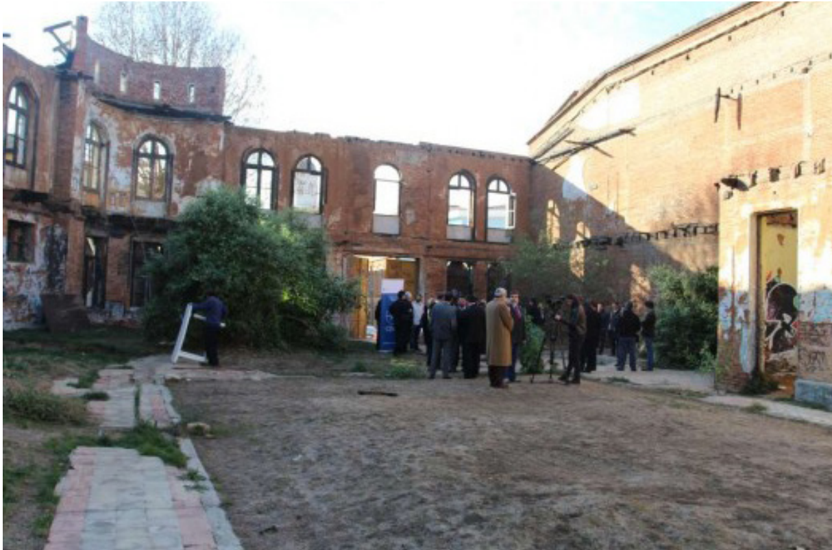
Site inspection at the Severin Building in decay
