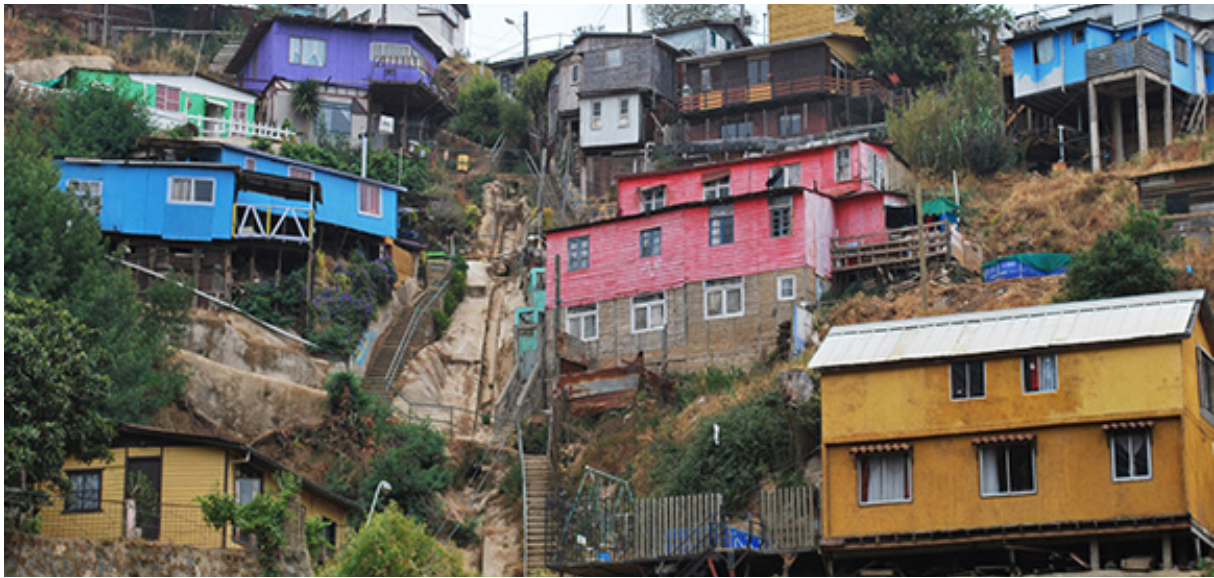
The fragmented, multi-level homes as a result of informal construction (Pino Vásquez & Ojeda Ledesma, 2013)
