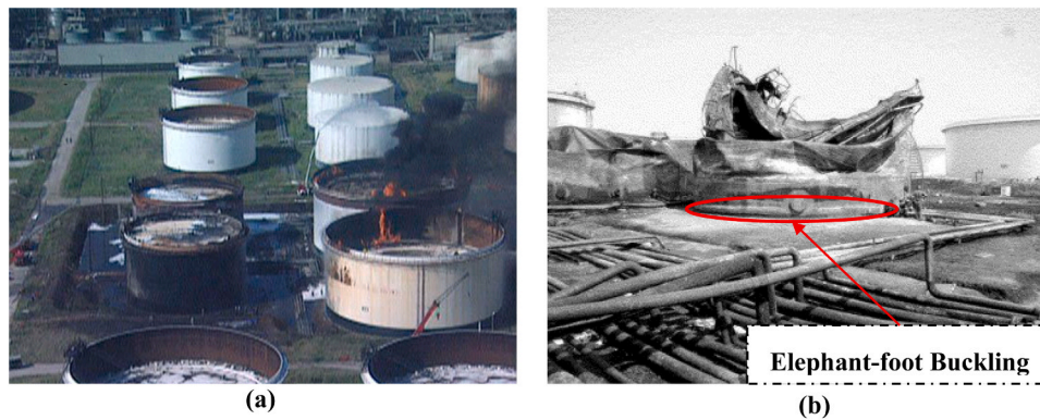
Fig. 1. Typical earthquake-triggered fire domino scenarios. (a) Massive fires at the TUPRAS Izmit refinery caused by 1999 Kocaeli earthquake (Girgin, 2011); (b) Tanks collapsed due to fires (Scawthorn and Johnson, 2000).
