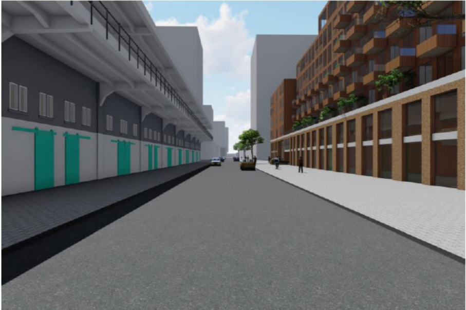
Option 1: Brick finishing for the plinth with Lunawood for the upper levels
