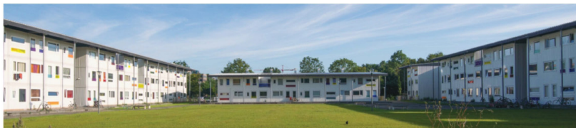
Startblock, Amsterdam, housing foundation De key
