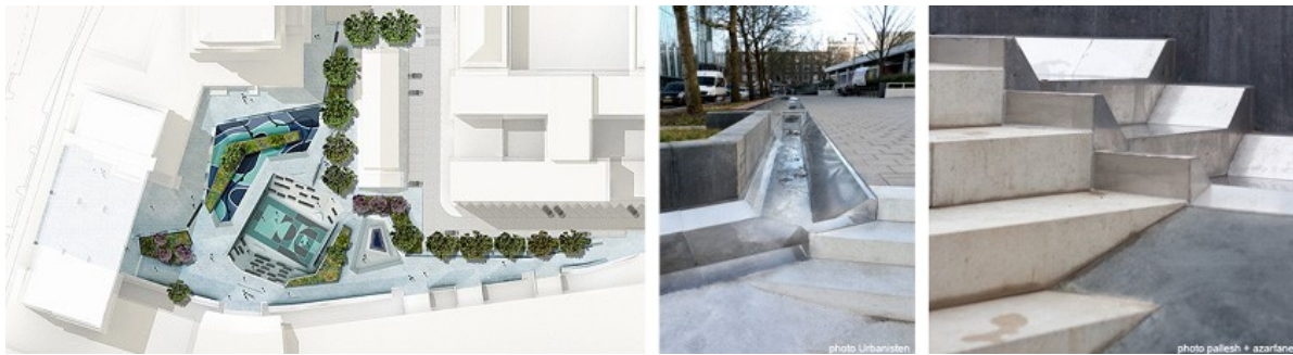
Figure 6.2: Benthem water square. Left: Overview of the design of the square. Middle and right: Steel gutters transport rainwater towards the basins. (De Urbanisten, 2013)
