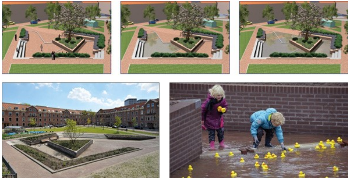
Figure 6.1: Bellamy water square. Above, the filling sequence during heavy rain (Gemeente Rotterdam, 2012). Below, photographs of the finished square (Straatbeeld, 2014)
