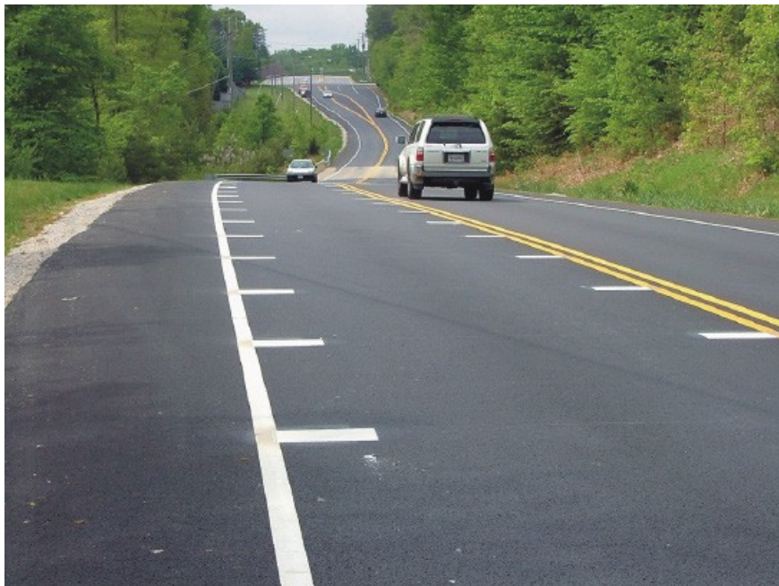
Figure 40. Peripheral speed reducing lane markings (FHWA, 2015)
