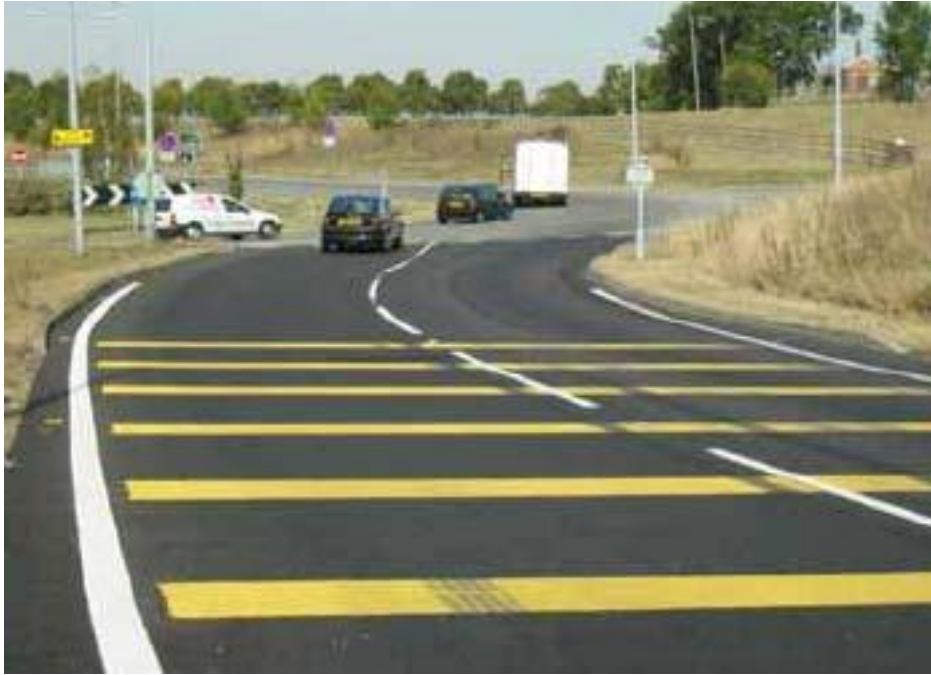
Figure 6. Transverse Lane Markings (Source: Google)
