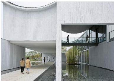
Figure 10: Community centre with water basin for rainwater harvesting (Detail, 2019).
