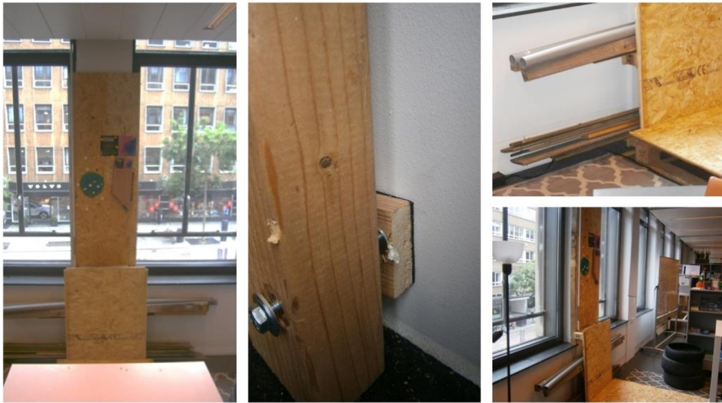
Figure 16. Wall design element. A vertical surface to attach things to without damaging the original wall. Clamped to the original wall.
