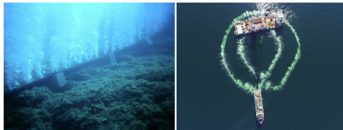
Figure 1.8: Air bubble cloud released by a perforated pile positioned on the seabed on the left. Double Big Bubble Curtain on the right(Tsouvalas, 2020). The air bubble curtains
