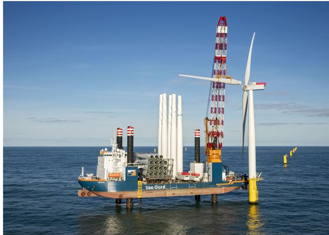
Figure 3.6: Rotor blade installation of 4 MW WTGs for the Gemini project (Van Oord, 2016)
