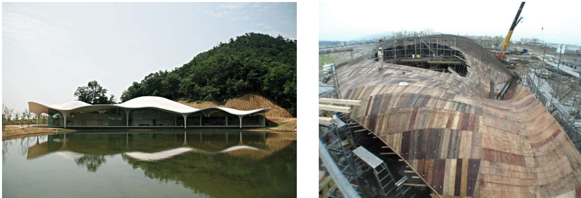
Figure 1-4: Meiso no Mori Crematorium by Toyo Ito and Associates, completed in 2006. a) Completed building b) Construction showing complex concrete formwork [12].
