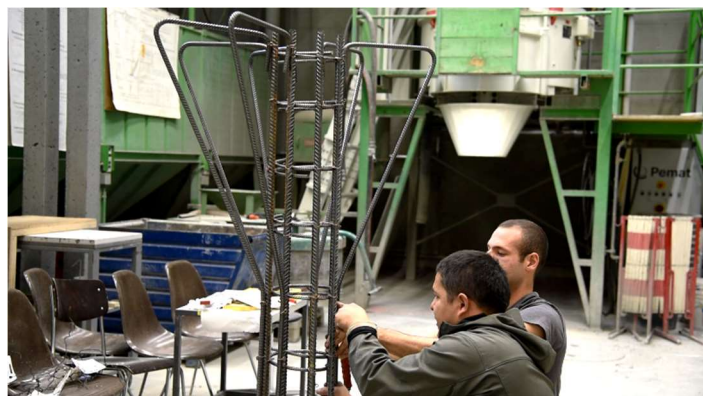
Figure 4-47: Assembly of reinforcement cage.
