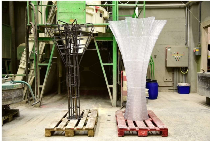
Figure 4-48: Completed prefabrication of reinforcement (left) and 3D printed formwork (right).
