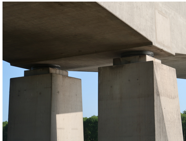
(b) The spherical bearings located at the intermediate supports.
