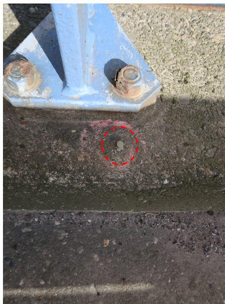
Figure 3.9: Brass bolt located on the deck of the Rooyensteijnse Brug.
