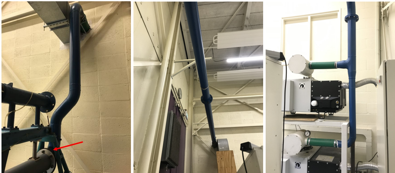
Figure 4.6: Full flow system from point of entrance at bellmouth to vacuum pumps no.1 and no.2. Images are not to scale.
