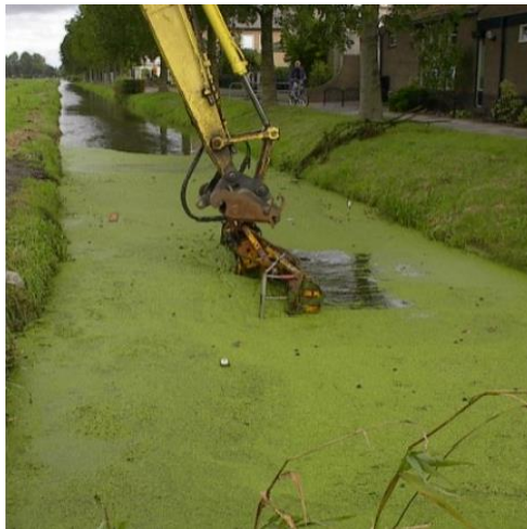
Figure 4.2a. and 4.2b. Wheeled excavator with dredge and wheeled excavator with flat sieve (Timmerman and Hoving, 2016).
