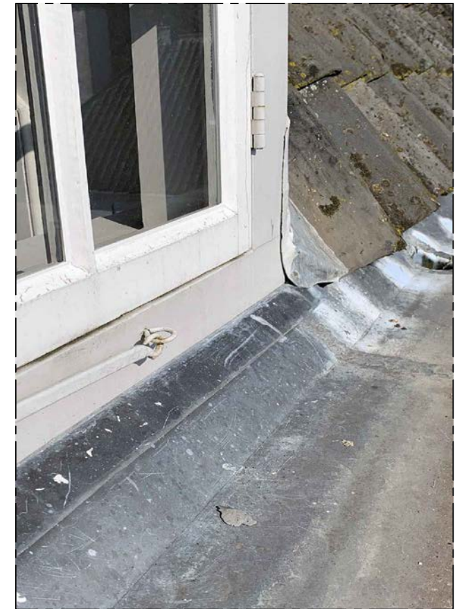
photo of dormer window and gutter
