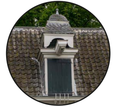
Wooden lifting hatch with slated roof
