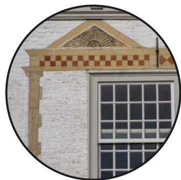
Wooden windowframes with sandstone ornamentation
