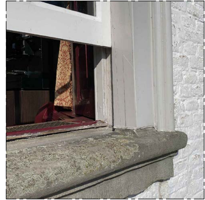
photo of window threshold
