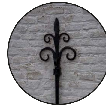
Wrought iron wall anchors
