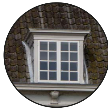
Dormers, combination of wood and plumbum
