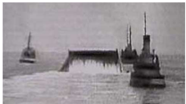
Figure A.1. The Pipe Lines Under the Ocean project (P.L.U.T.O.), to the left the large conundrum to which the pipe was wound, to the right the tugs which were used to roll out the pipe as it was laid across the English Channel (Source: [15])
