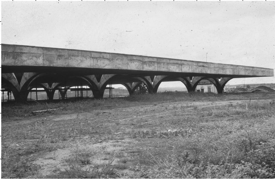
Jaú's bus terminal under construction, 1973, architect João Vilanova Artigas. Source: Faculty of Architecture and Urban Planning Library, University of São Paulo in: www.arquigrafia.org.br/photos/1096 cc-by-nc-nd
