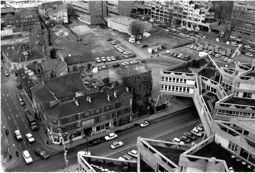
Jean Renaudie, Jeanne Hachette mixed-use complex (1969–75), Ivry-sur-Seine, France. Courtesy of Archives municipales d'Ivry-sur-Seine.
