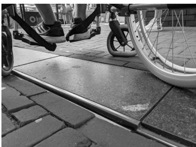
Fig. 2.4 (by author): ‘(Small) gutters are problematic for the wheelchairs’ wheels. They could get stuck or the rubber tire itself could come off, probably resulting in a situation the user can not solve on its own.’
