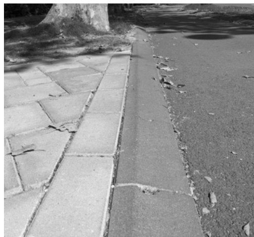
Fig. 2.1 (by author): ‘Quickly noticeable was that even the smallest hill or threshold can be annoying for a wheelchair user, especially if it is too steep. The power that is needed to push that last bit is quite big, which elderly persons can often no longer produce at their age.’
