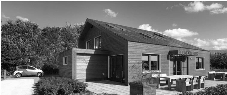
FIG.7.2 ECONEXIS DEMO HOUSE IN ZWOLLE. THE HOUSE IS BUILT TO LOOK LIKE A HOUSE WHERE PEOPLE CAN SEE THEMSELVES LIVE. INCLUDES ALL MODERN ENERGY TECHNOLOGY, WHICH ARE HARDLY VISIBLE
