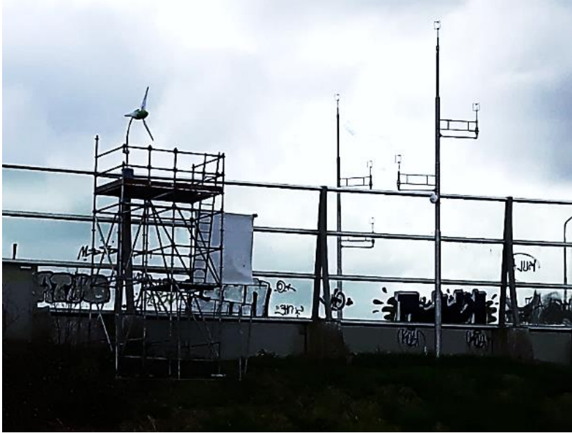
Figure 3 - 7 : Micro wind turbine integrated on noise barrier field experiment. The 6 sonic anemometers are visible on the right located on two masts on three heights. The scaffolding behind the barrier is for access purposes and does not influence the incoming flow over the barrier.
