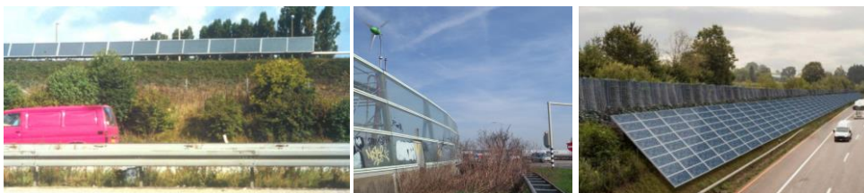
Figure 4 - 1: Different types of noise barriers (left) earth embankment type of Photovoltaic Noise Barrier [24] (middle) acoustic screen type of micro wind turbine noise barrier (right) combination of an earth embankment photovoltaic noise barrier with an acoustic screen [25]
