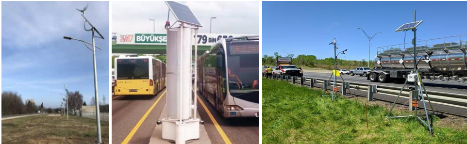
Figure 1-4: Concepts and research of wind energy along highways and turbines integrated with highway infrastructures (left) light pole mounted horizontal axis wind turbine next to a road, (middle) vertical axis wind turbine installed on top of a median of a highway and (right) experimental set-up of wind energy generation along North Carolina's highways
