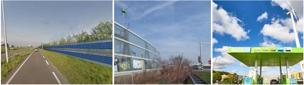
Figure 1-2: (left) photovoltaic noise barrier PVNB, (middle) micro wind turbine noise barrier (MWTNB), (right) wind powered hydrogen producing refuelling station concepts
