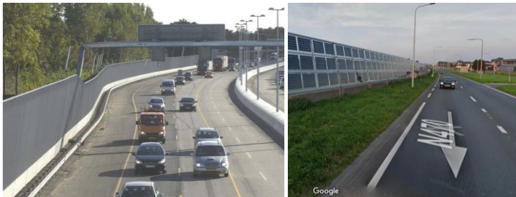
Figure 4 - 2: Photo examples of noise barrier tilt orientation (left) noise barrier with a forward tilt towards the road [24] (right) noise barrier with a backwards tilt towards the road
