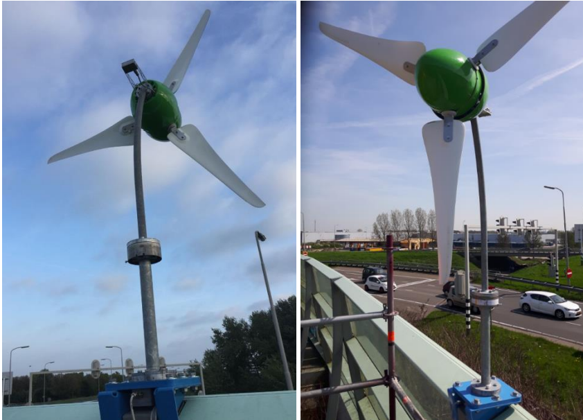
Figure 3 - 1: Micro wind turbine integrated on top of the noise barrier.
