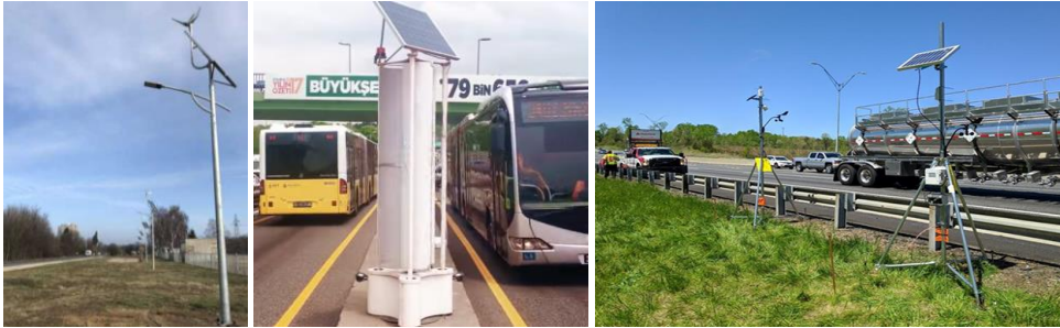
Figure 5 - 2: Concepts and research of wind energy along highways and turbines integrated with highway infrastructures (left) light pole mounted horizontal axis wind turbine next to a road, (middle) vertical axis wind turbine installed on top of a median of a highway and (right) experimental set-up of wind energy generation along North Carolina's highways
