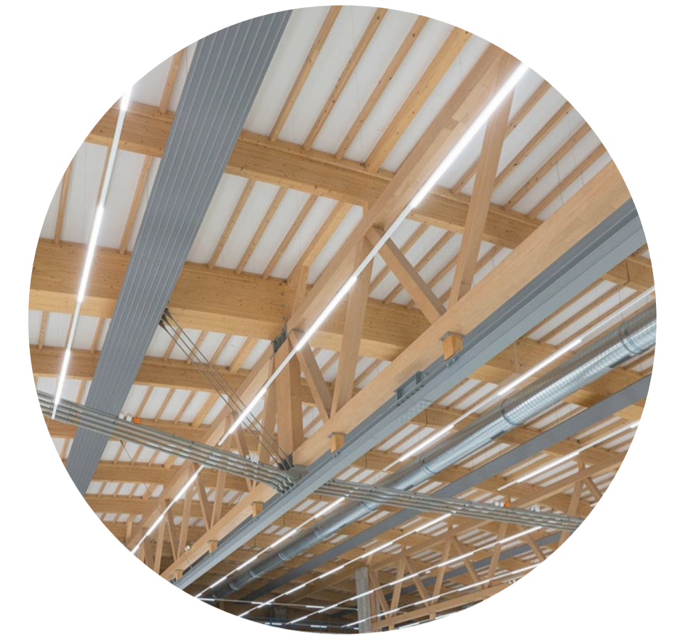
reference - hybrid wood-steel tension construction
