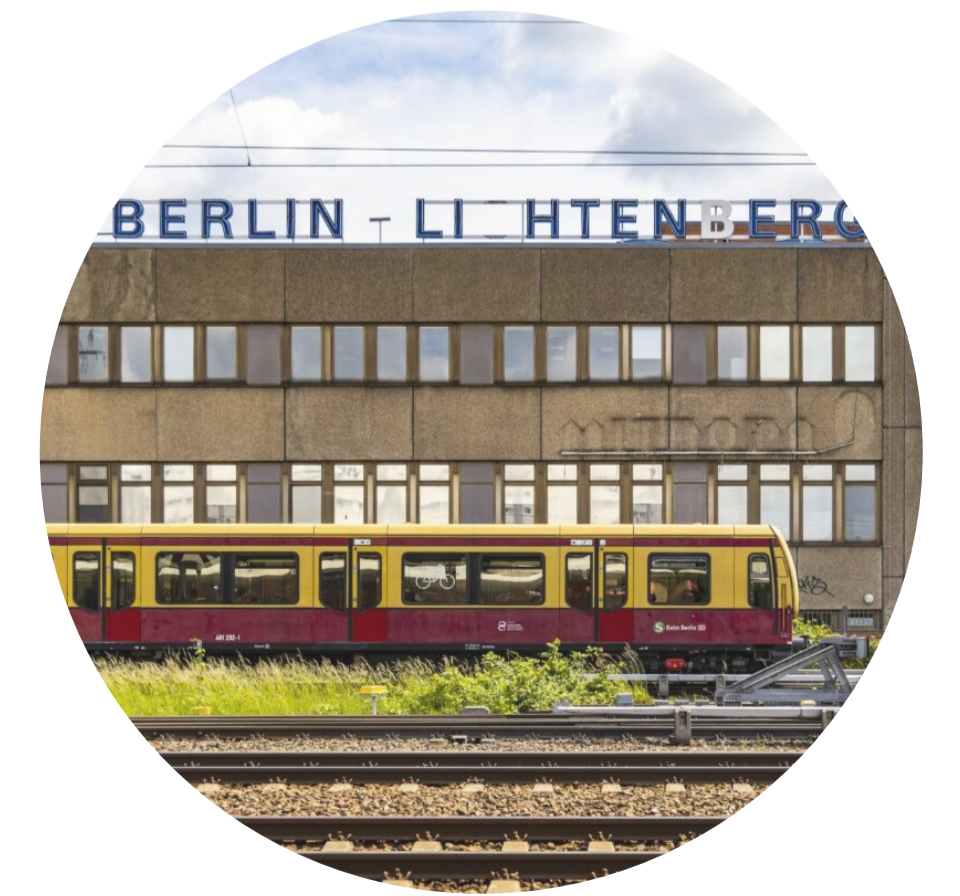
existing concrete station building to be re-used
