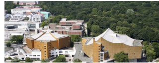
Construction of the Arts and crafts museum by Rolf Gutbrod
