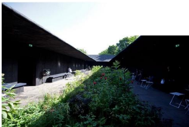
Pic11 Serpentine pavilion by Peter Zumthor. Corridor of the labyrinth, central garden and plan of the structure.
