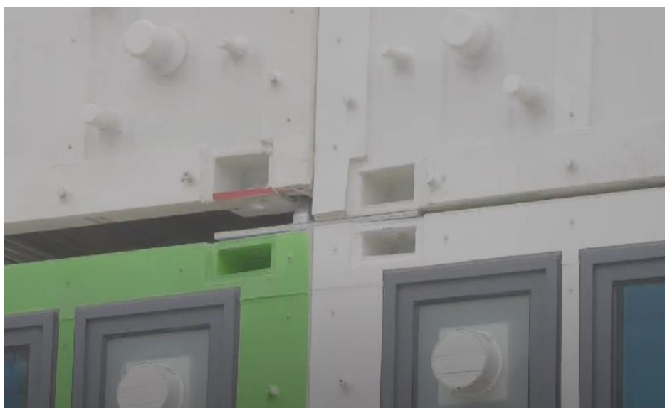
Figure 29. Inter-module connection (CIMC Modular Building Systems, 2022)
