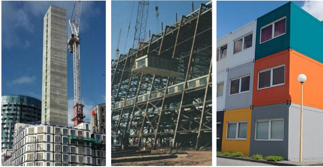
Figure 11. Core structure, frame structure and self-supporting structure (Thai et al., 2020; Falcon Structures)
