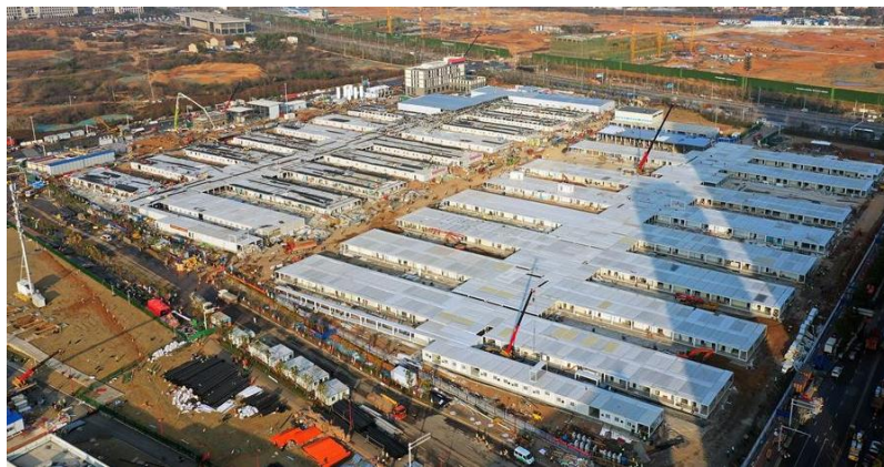
Figure 25. Leishenshan Hospital under construction (the Design Museum, 2020)
