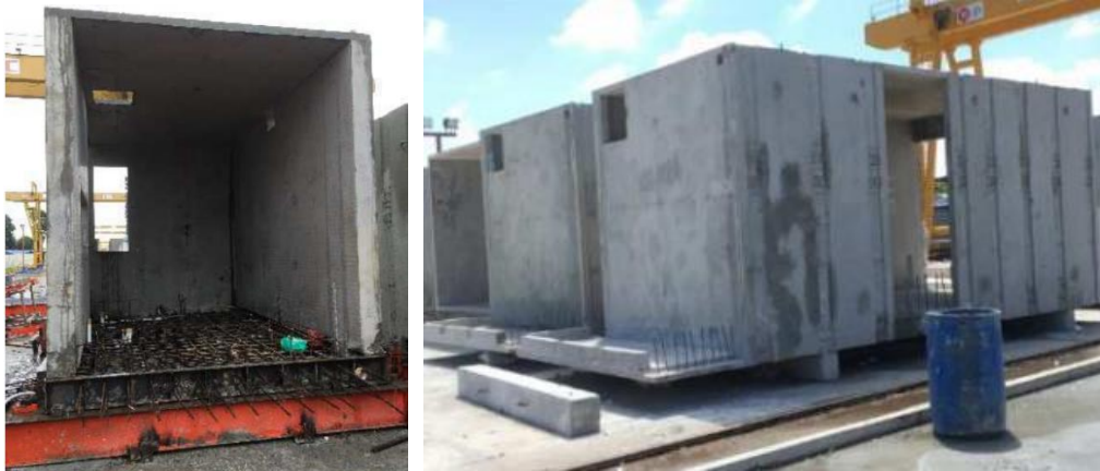
Figure 15. Module in production and after completion (Seng et al., 2021)
