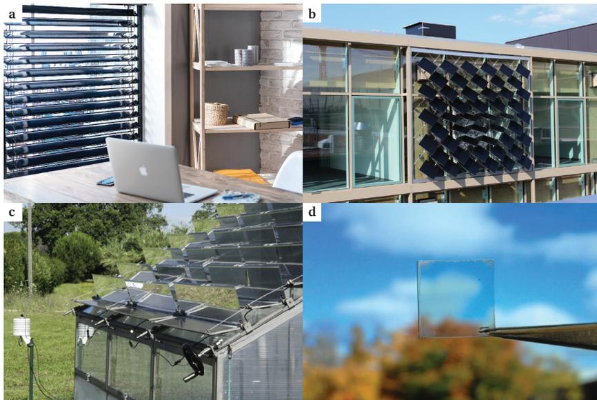
Figure 1.6: Existing PV-window demonstrations. **a**, Smart solar blinds from SolarGaps. **b**, Adaptive solar façade at the House of Natural Resources [27]. **c**, PV greenhouse with reflective aluminum mirrors [28]. **d**, Transparent PV solar device [29].
