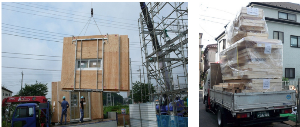
Figure 3: Pre-assembly at Factory (left) and Assembly at Construction Site (Right)
