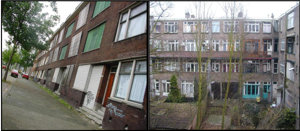
Figure 1: picture Wallisblok before renovation (2004)
