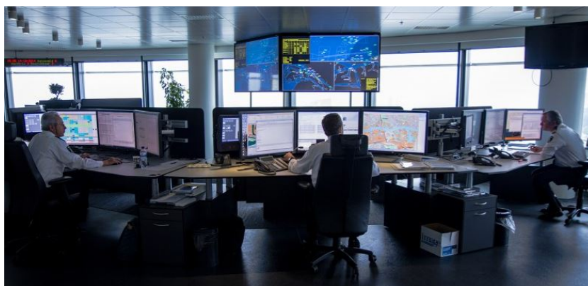
Figure D.3: Harbour Coordination Center [conducted from schuttevaer.nl]
