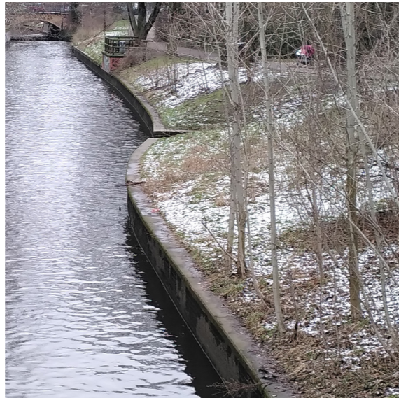
Figure 4.5d. Low wall with vegetated bank
