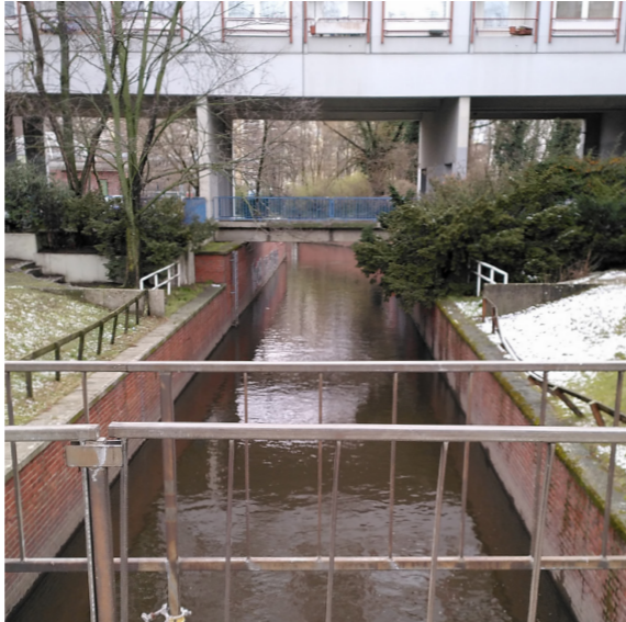
Figure 4.3d. Building above the water
