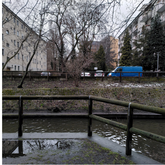
Figure 4.5b. Wall with stone bank
