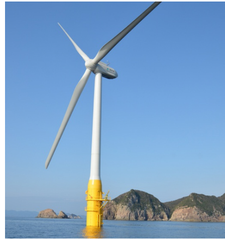
(b) Hitachi 2.1 MW wind turbine used in the Goto City Wind Farm [62]
