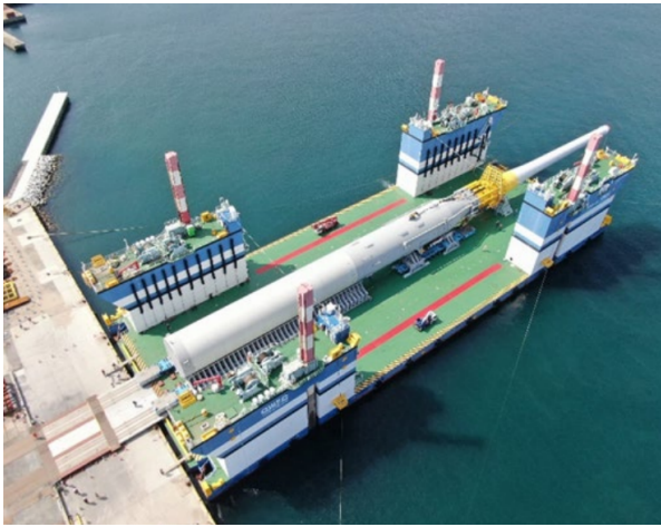
(a) Deployment of the first SPAR-buoy floater used for the Goto City Wind Farm [94]
