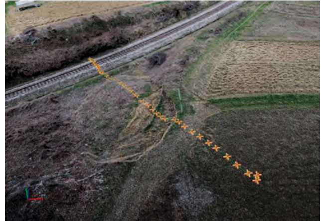
Fig. 3. Drone application for the determination of railway slope cross-sections
