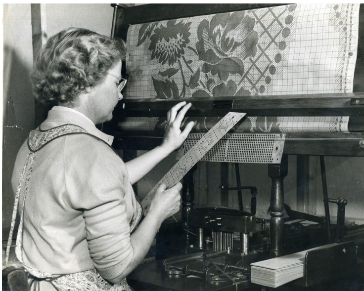
Card maker using a machine to translate a pattern onto punch cards, c. 1950.
