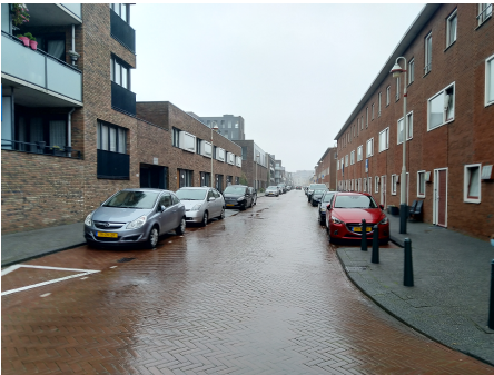
Figure F.1: Typical Duindorp street
