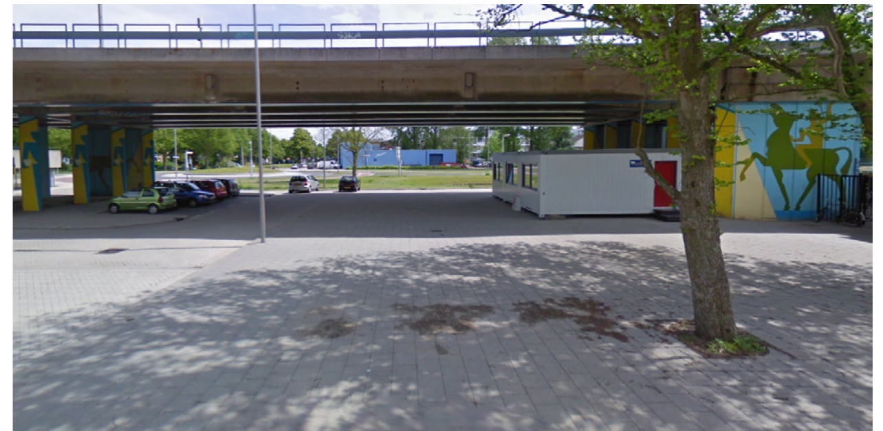
Pic 6.3.1.3 Current condition of design interventio area
