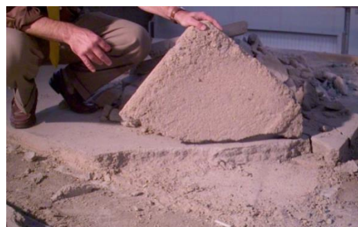
Figure 6-30: Removing the cement floor from a hollow core slab (Buunk & Heebing, 2017)
